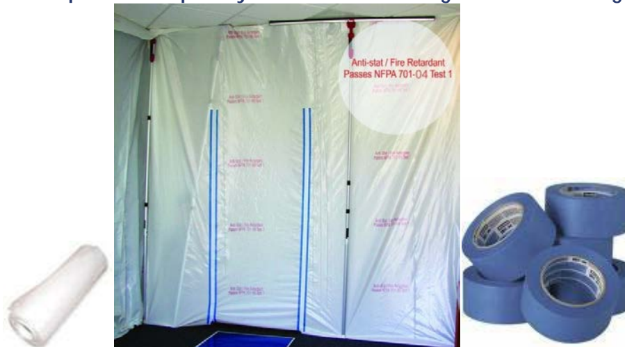
Figure 5: Example of Temporary Containment Using Plastic Sheeting and Tape
