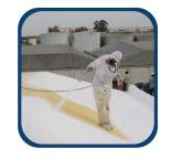
GCMC Ultra-Thane 230 roof foam will improve a building's energy efficiency by providing a continuous thermal break from its uniform layer of 6.5 per inch "R" value insulation. Ultra-Thane 230 roof foam used in conjunction with our reflective roof coatings provides maximum economic benefit to keep your building cooler in summer and warmer in winter.
