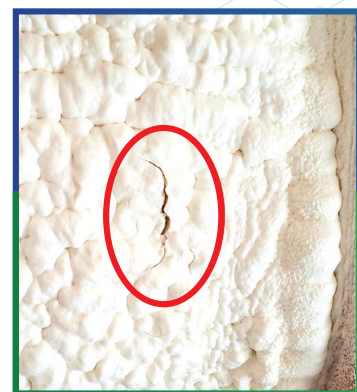
2.0 Max sprayed at 3.5" thick in August
